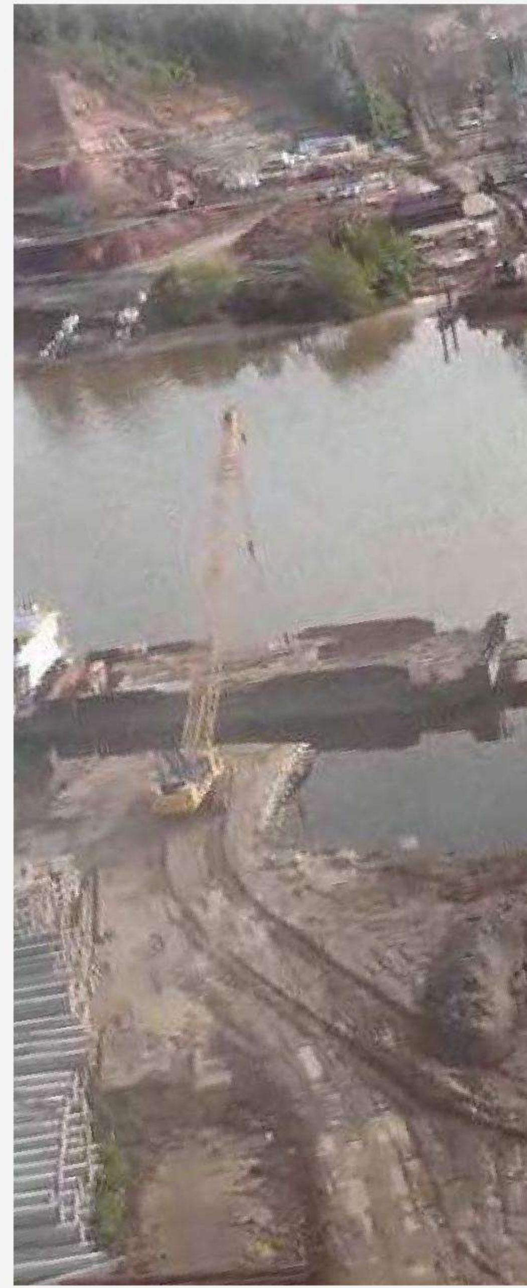
Limbang Bridge - Serawak, Malaysia
