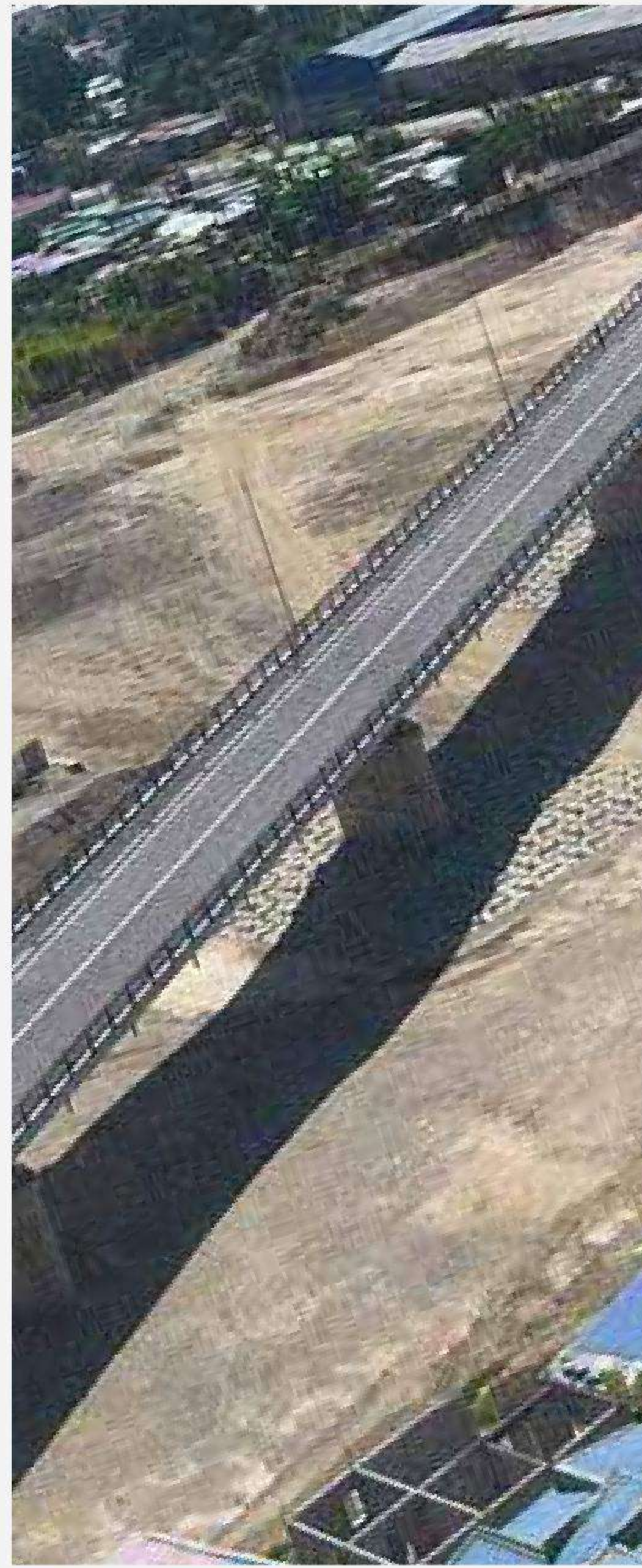
Comoro Bridge - Dili, Timor Leste
